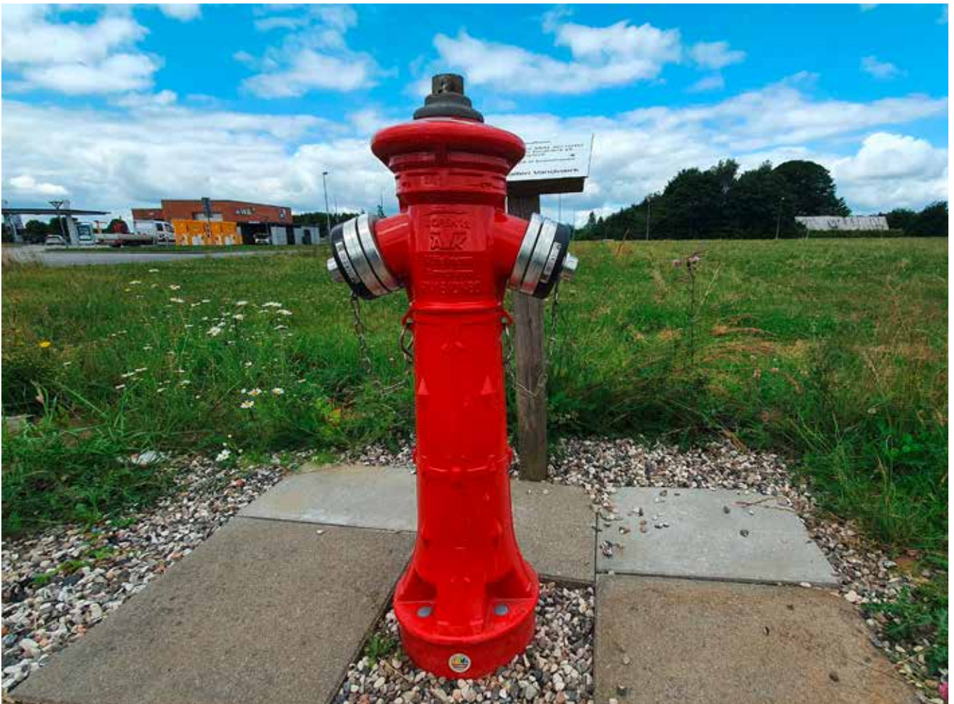
Hydrant with VIDI Caps installed. The use of a hydrant affects the pressure in an area. Therefore, it is important for the utility to know when the hydrant is being used in order to distinguish between a pressure drop coming from regular use or from a pipe burst.
